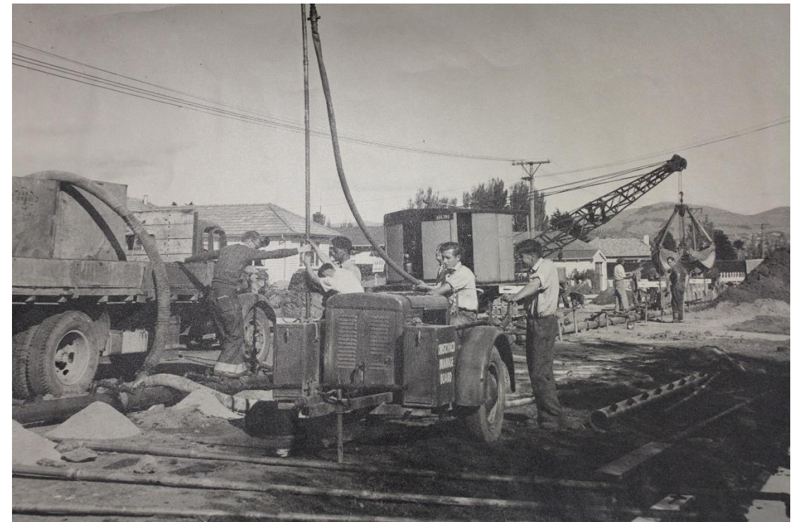
Christchurch Drainage Board – street sewer construction c.1950s
